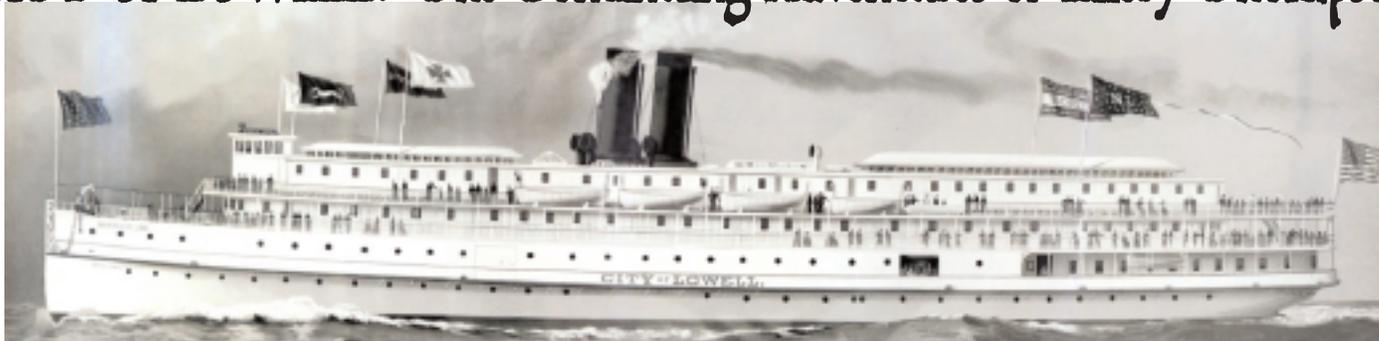
*City of Lowell (Hull 8) Passenger Steamer for the Norwich and New York Transportation Co., Length: 322'-4", Beam: 49'-6", Draft: 13' Launched November 21, 1893. Used between New York and the Eastern end of Long Island Sound until approximately 1935.*
